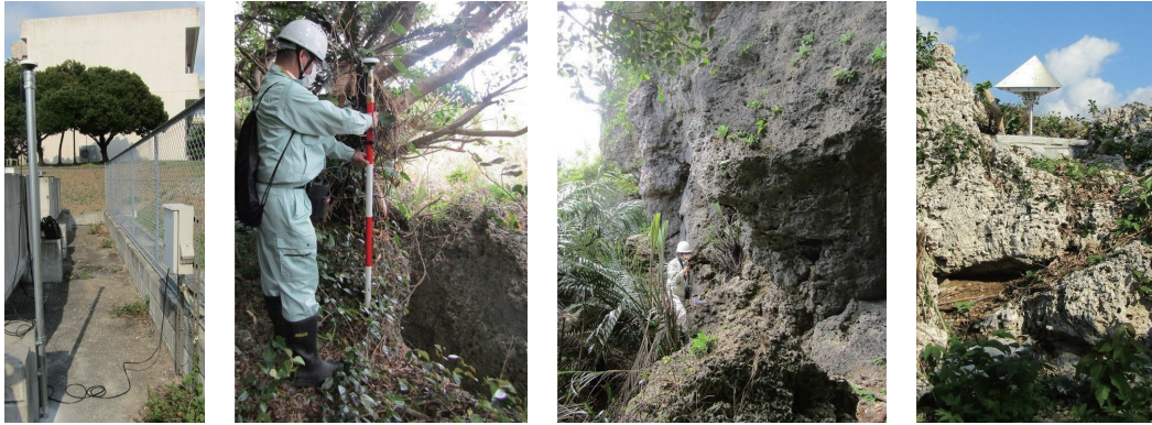
A. RTK B. Crack mapping C. Laser Scanning of the cliff D. Marker
