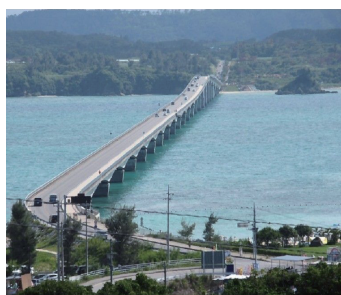
A. A view of the Kouri Bridge.
